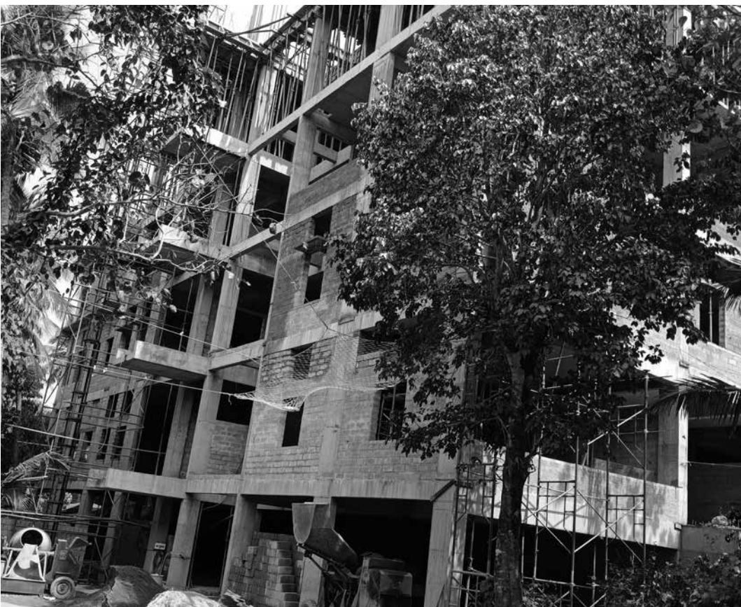
The New Library Complex under Construction
