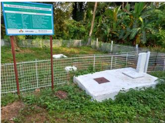
ECOSAN Biogas plant was installed in the hostel for effective disposal of human excreta. Capacity of the plant is 50m<sup>3</sup>. One more Biogas plant was installed in the carmel hill convent in the campus.
