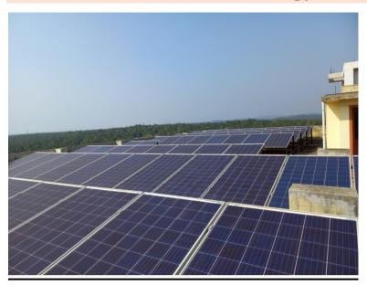
30KW on grid solar power plants are installed in the campus under CPE fund. solar power plant was connected to distribution system of Kerala electricity board from 2018 onwards.
