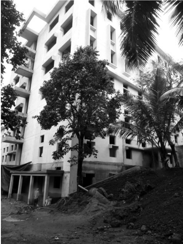
The New Library Complex under construction
