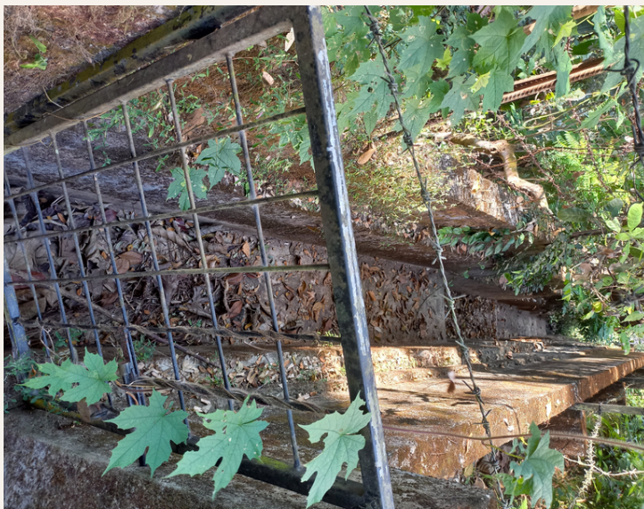
Rain Water harvesting pit Surface water flows down to the harvesting pit and is restored as the ground water.
