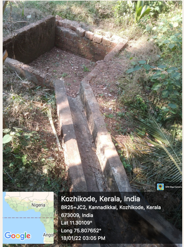
Rain Water harvesting pit Surface water flows down to the harvesting pit and is restored as the ground water.
