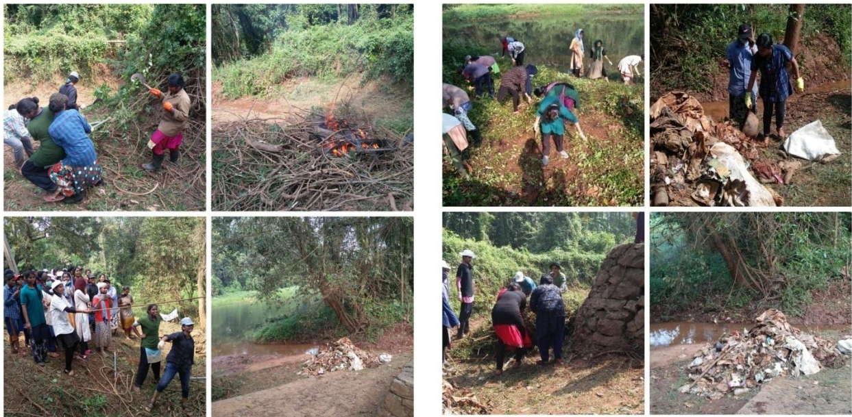
Cleaning work in Progress
