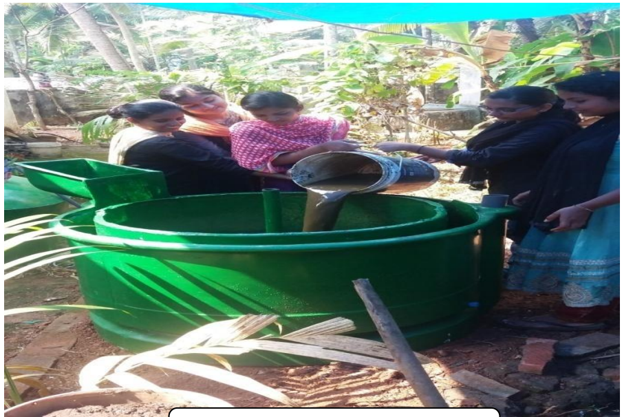
Biogas Plant Installation
