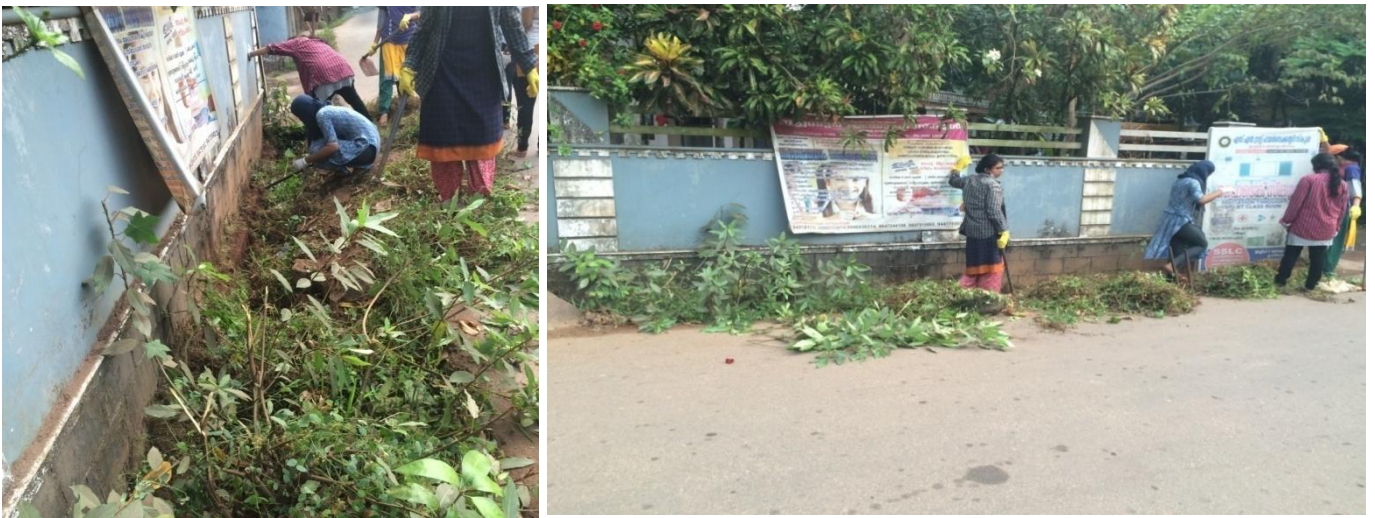
Cleaning the drainage at Ichannur
